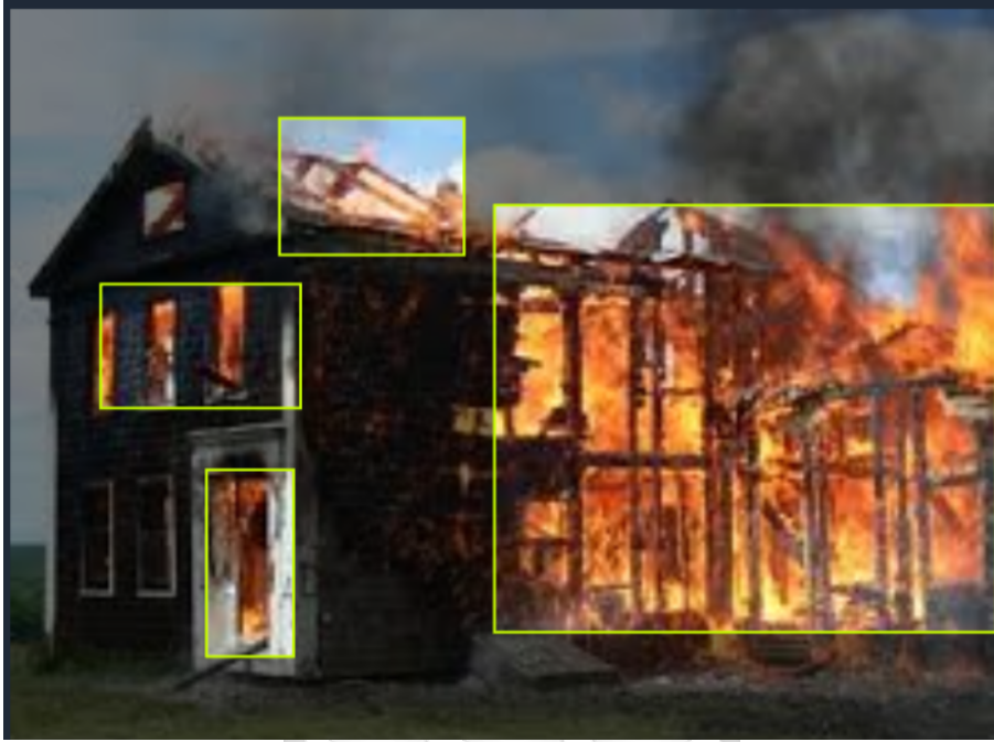
Figure 3.2: Fire hazard image used for training, hazard enclosed by yellow bounding box
