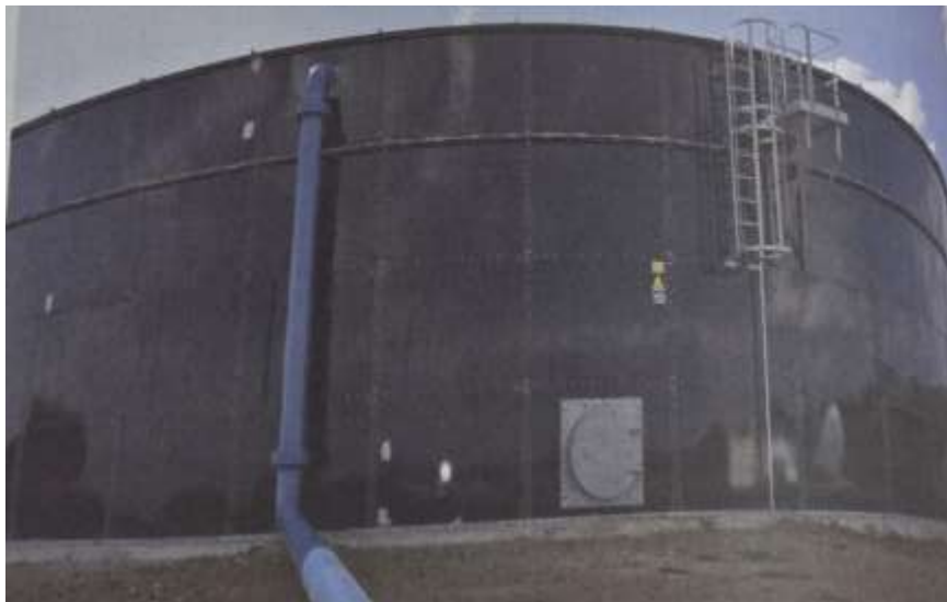
A GDC 4million liters water reservoir (Source: Field Data, 2025)
