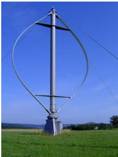
Fig. 3: Vertical axis wind turbine
