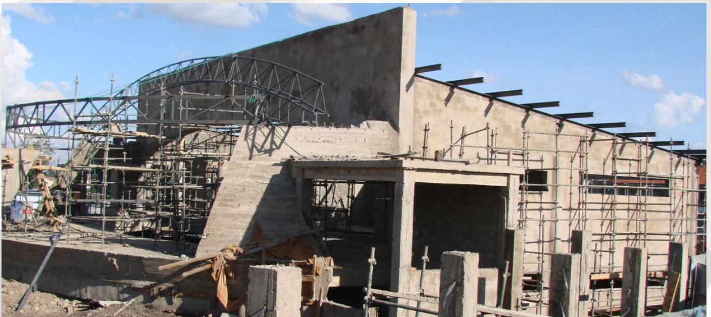
The SBS Building under construction
