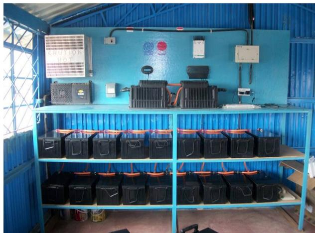
Figure 3 - Power House showing the controllers and Battery Bank
