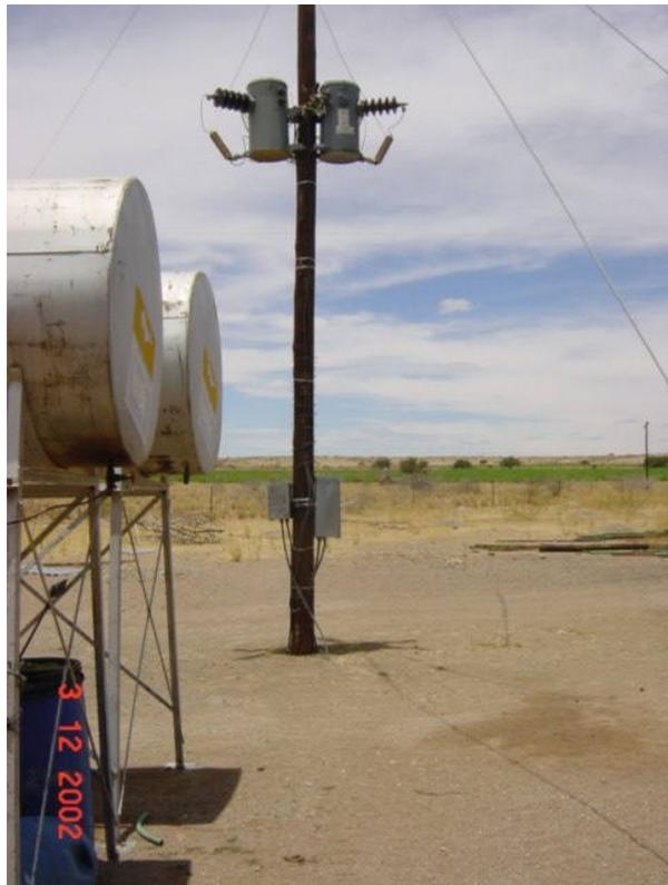
32kVA in parallel to a 48 kVA transformer – irrigation project, 3 phase submersible pump powered via a 11kVA converter drive
