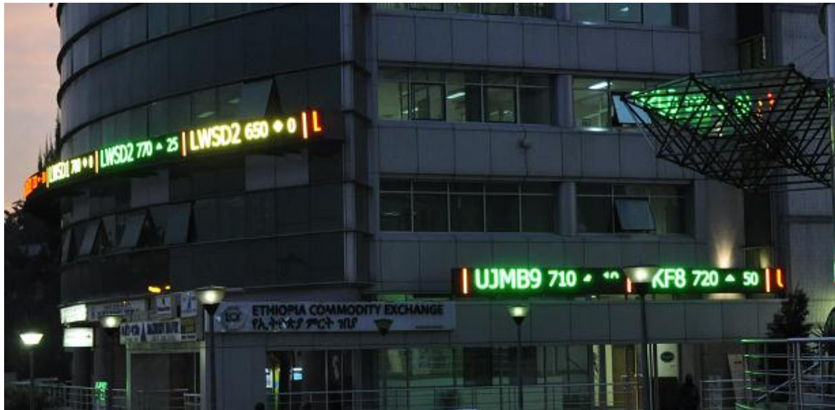
Figure H. 1 Electronic Tickers on ECX building
